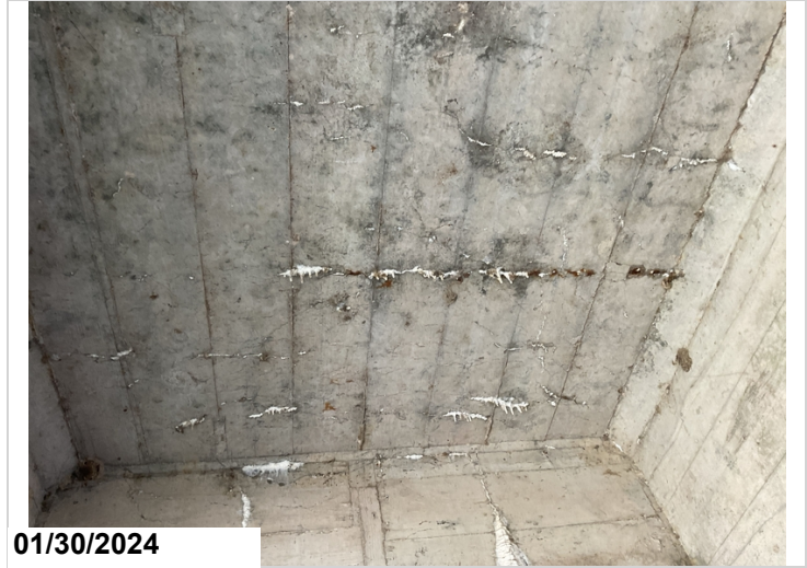
Efflorescent cracking with rust stains to soffit @ Span 5.(#3)
