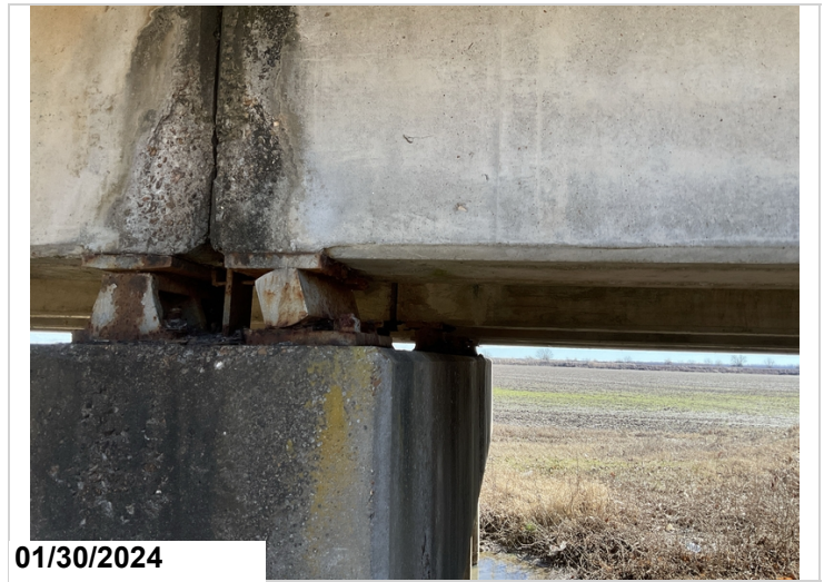
Moveable Bearings @ Bent 1 have rotated ahead.
