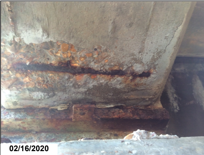
Span 10. Girder 4 has spall with 10" exposed rebar at beginning of span.
