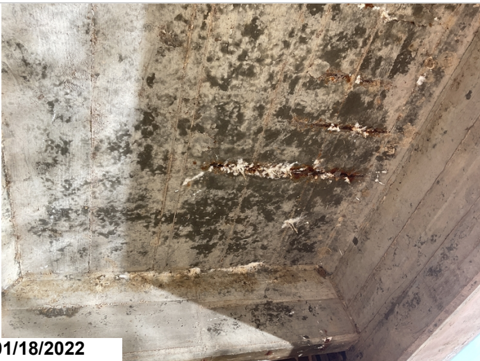
Efflor cracks to soffit between girders 3 & 4 @ end of span 9.
