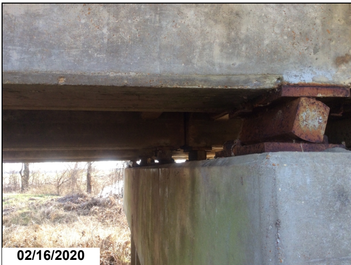
Bearings have rotated to limits and no longer function @ Bent 9.
