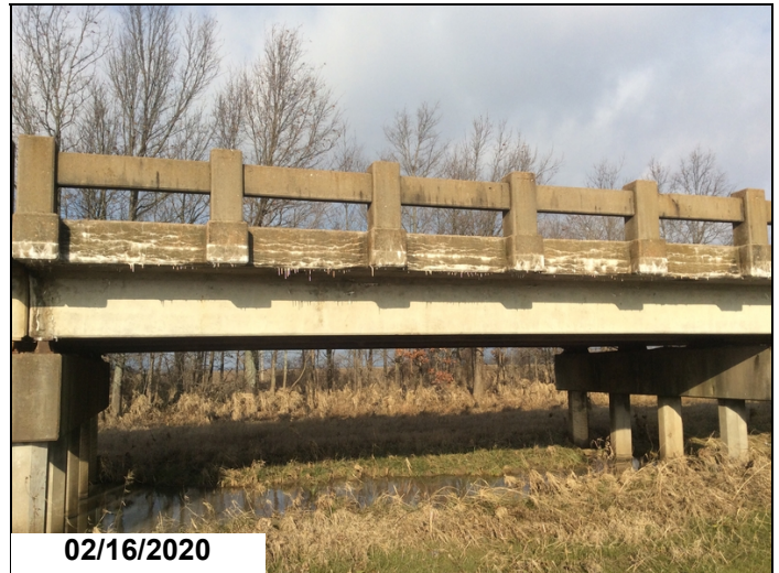
Span 3 Right. Severe map cracking with efflorescence to outside of deck.
