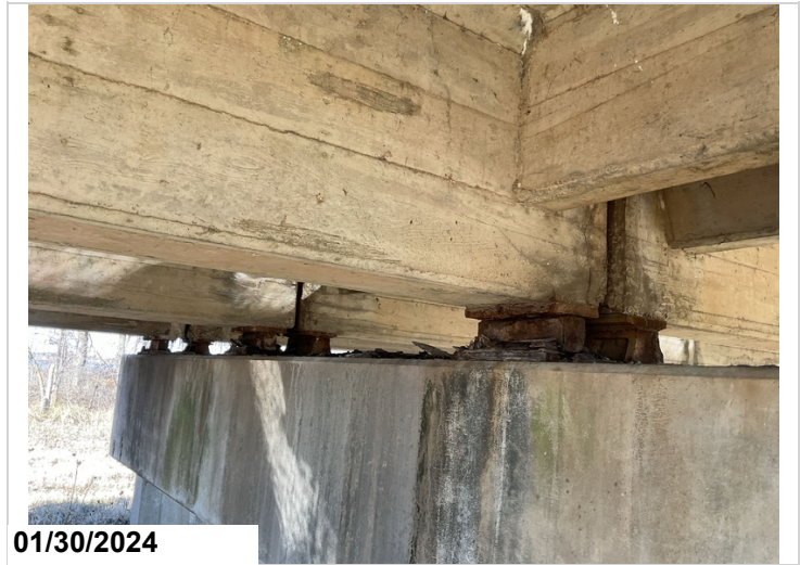
Rust with pack rust to Moveable Bearings 2 & 3 @ Bent 5. (#3)
