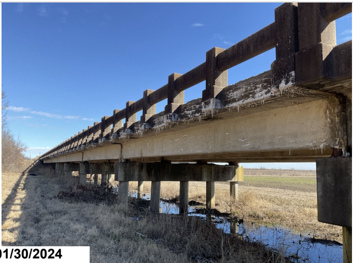
Heavy efflorescent map cracking to Left outside edge of deck @ Spans 3 - 7.(#3)
