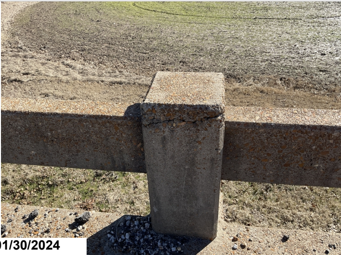
Typical cracking to Concrete Posts.(#3)
