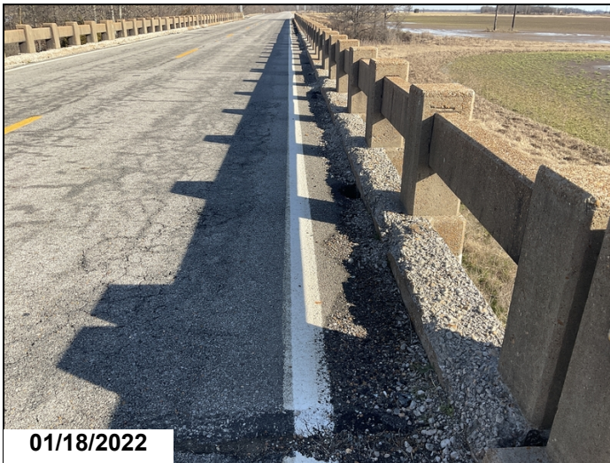
Curb: Left and Right Sides of Spans 3 through 9 are deteriorated and spalled.
