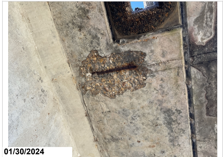
Spall with rebar exposed with s/l to 2nd drain opening on Left @ Span 1.(#3 typical)
