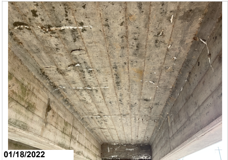
Typical efflor cracks to soffit @ all spans.
