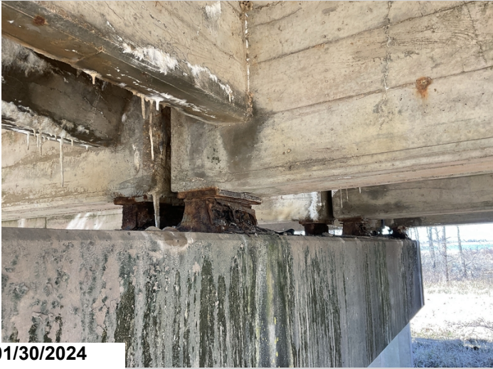
Rust with pack rust to Fixed Bearings @ Bent 4.(#3)
