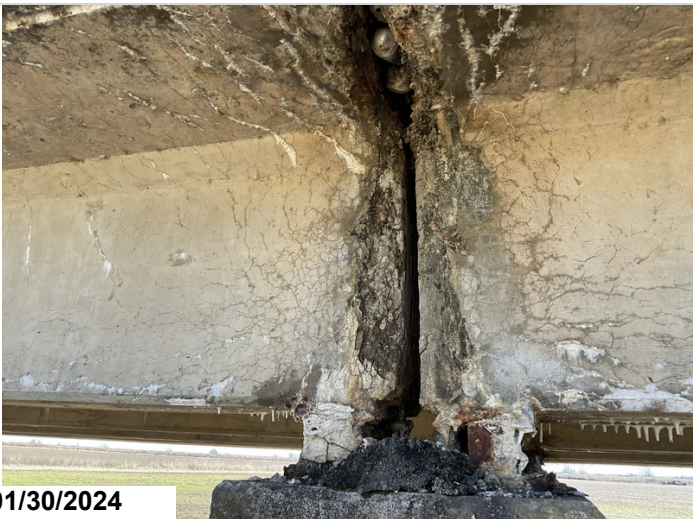
Spalls to Girder 1 @ Bent 4.(#3)
