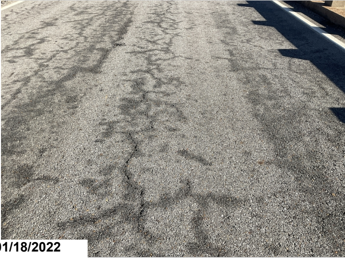
Typical cracks to wearing surface @ all spans.
