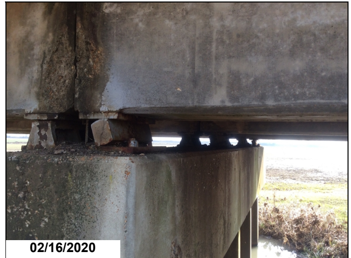
Bearings have rotated to limits and no longer function @ Bent 1.
