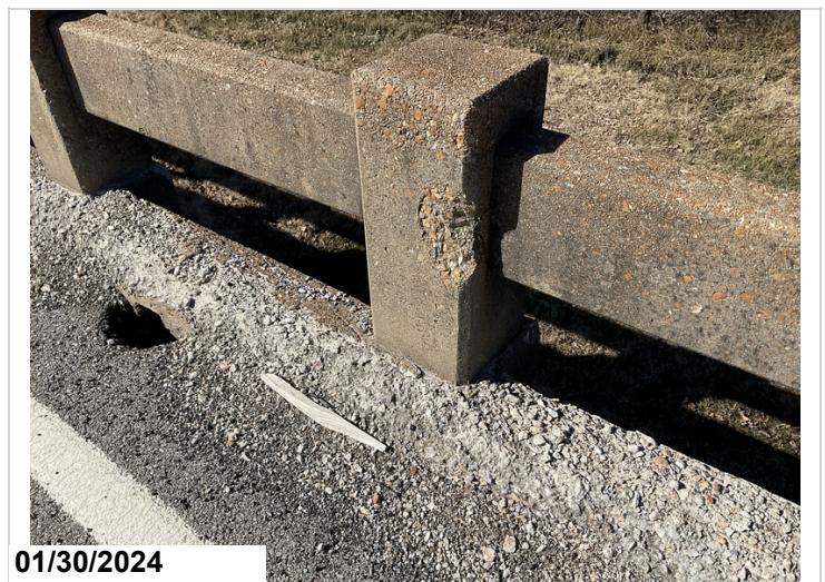
Typical spalling to Right bridge rail.(#3)
