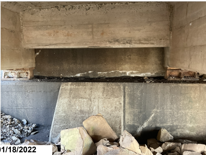
Efflorescent cracks to backwall @ Abutment 2.
