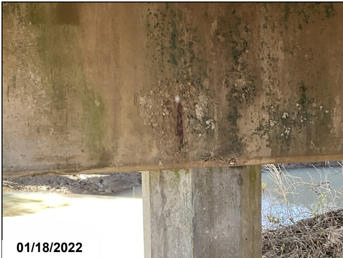
Concrete Caps all Bents Spalls with exposed rebar.
