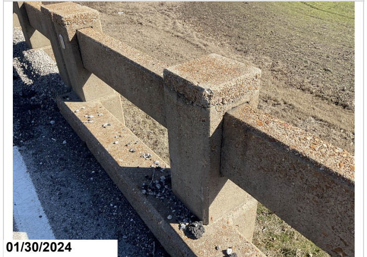
Typical cracking to Concrete Posts.(#3)
