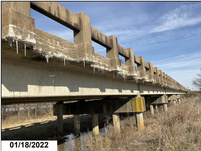
Spans 1, 3,4,5,6,7,8,&9 Outside Edge of Deck has Severe Efflorescent Map Cracking.
