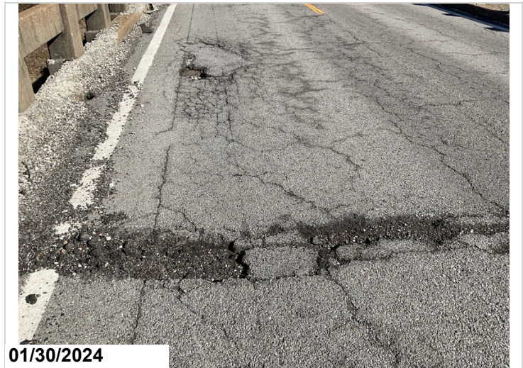
Spalls/potholes in asphalt overlay @ Bent 5 & Span 6.(#3)
