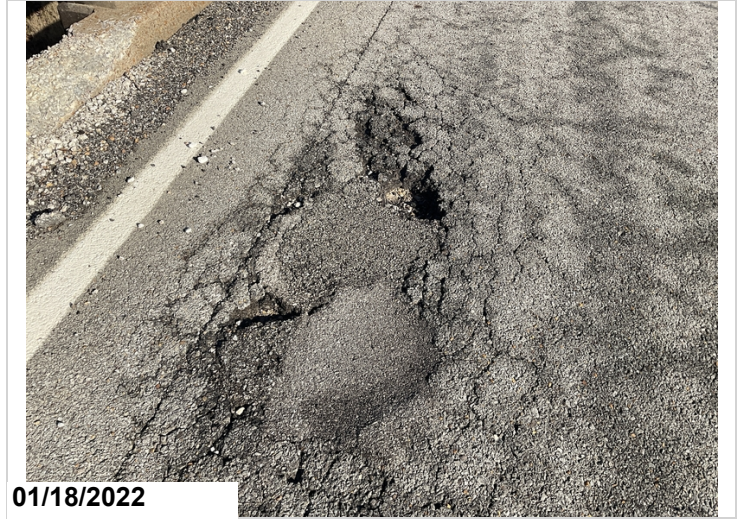
Potholing to joint & asphalt overlay in Left lane @ Span 6.
