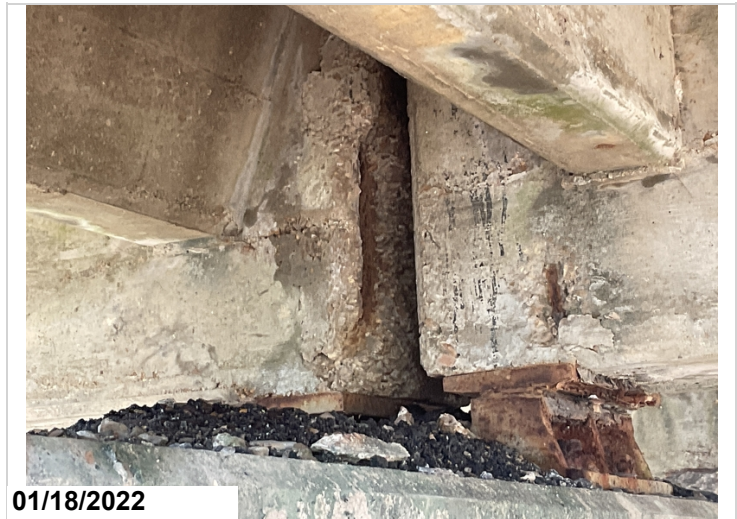
Spall with rebar exposed to back of girder 3 over bent 3.
