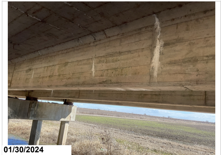
Efflorescent cracking to Girder 2 @ Span 5.(#2)
