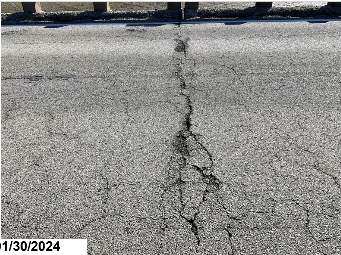
Typical debris impactation to Assembly Joint.(#3)
