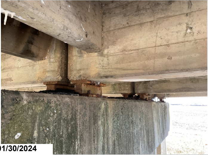
Light rust to Moveable Bearings 2 & 3 @ Bent 3.(#2)
