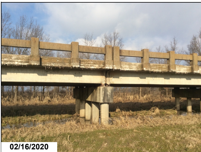
Spans 4 & 5 Right. Severe map cracking with efflorescence to outside edge of deck.
