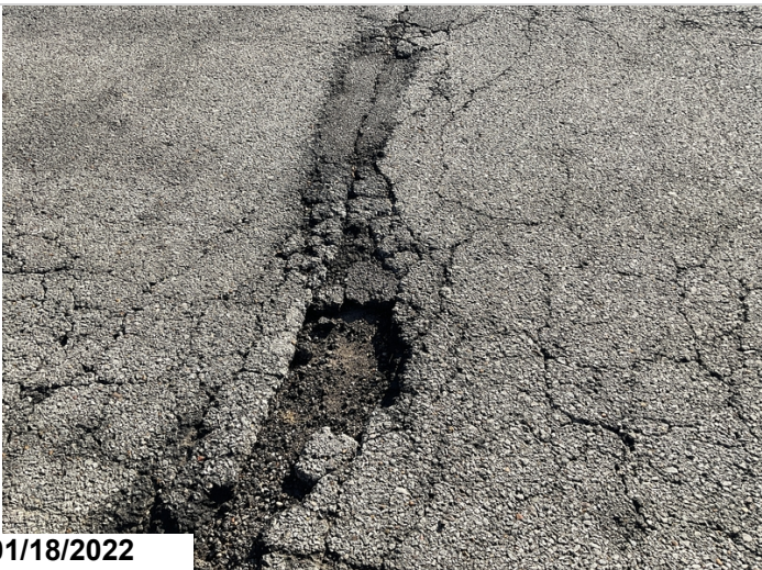
Typical spalls to joints @ all spans.
