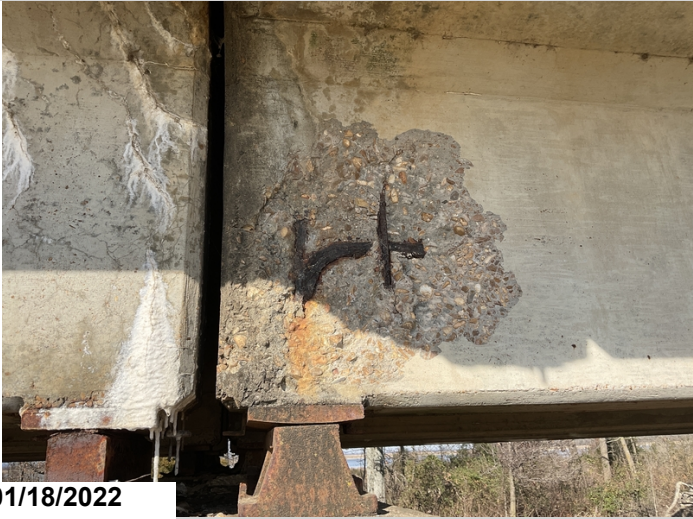
Spall with rebar exposed to girder 4 @ beginning of span 8.
