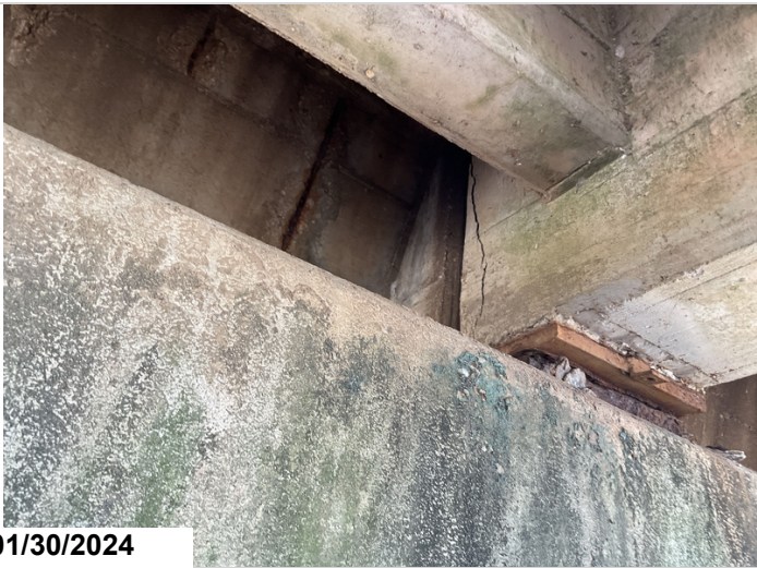
Large crack to end of Girder 3 @ end of Span 7(#3)
