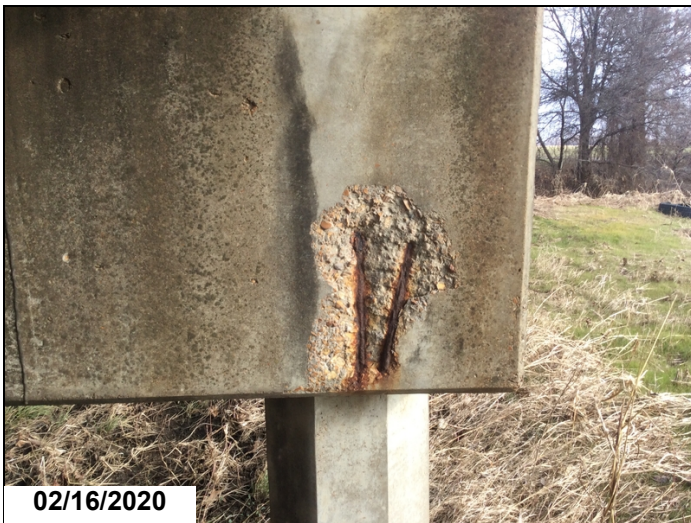
Spall with 24" rebar exposed to Right side of cap @ Bent
