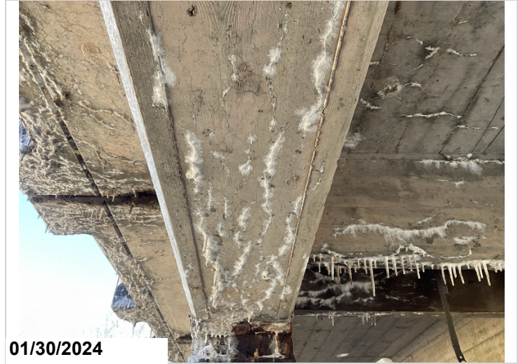
Efflorescent map cracking to bottom of Girder 1 @ Span 3. (#3)
