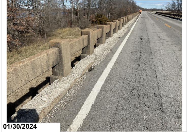
Typical spalling to Left curb.(#3)
