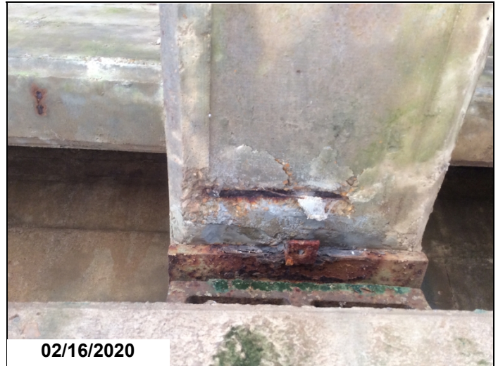
Span 2. Girders 3 & 4 have 6" Spall with 6" rebar exposed to bottom at beginning of span.
