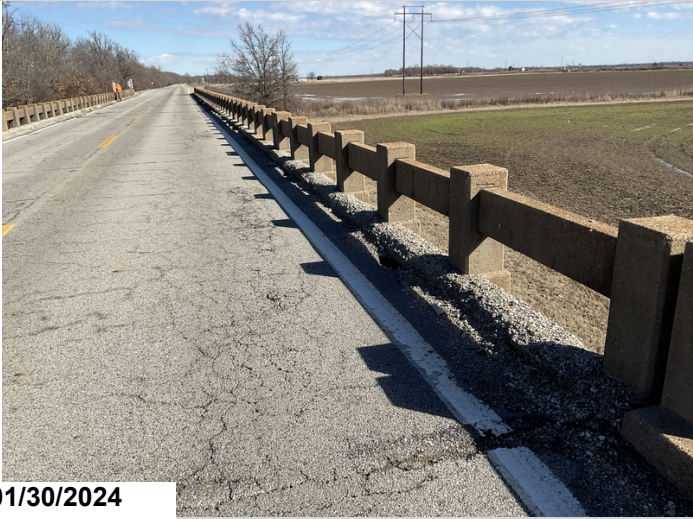
Typical spalling to Right curb.(#3)
