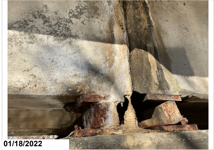
Efflor crack to girder 4 @ end of span 9.
