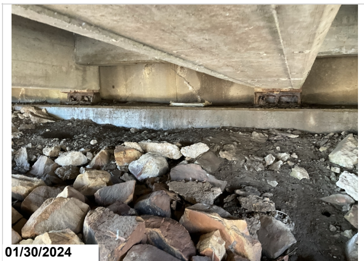
Rust with pack rust to Fixed Bearings @ Abutment 1.(#3 typical)
