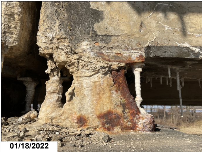
Bents 1 and 9 under all Girders. Bearings have rotated to limits and no longer function.
