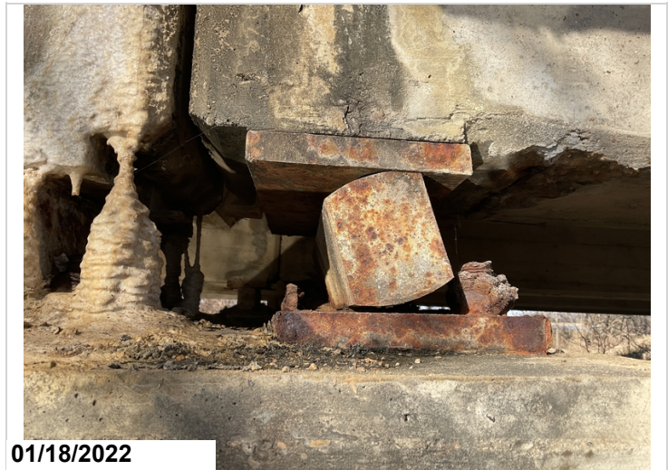
Moveable bearing has rotated back @ Bent 9.
