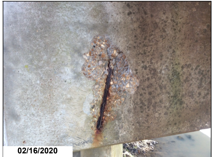
Spall with 12" rebar are exposed to Left side of cap @ Bent 1.
